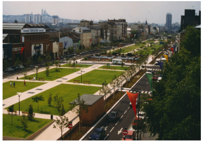
REF: Couverture de l'autoroute A1, Paris, France
